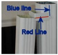
Screw should be installed at a horizontal even or just above the height of the extension end when raised up. See Red line, and vertical position in center of downspout, Blue line.
